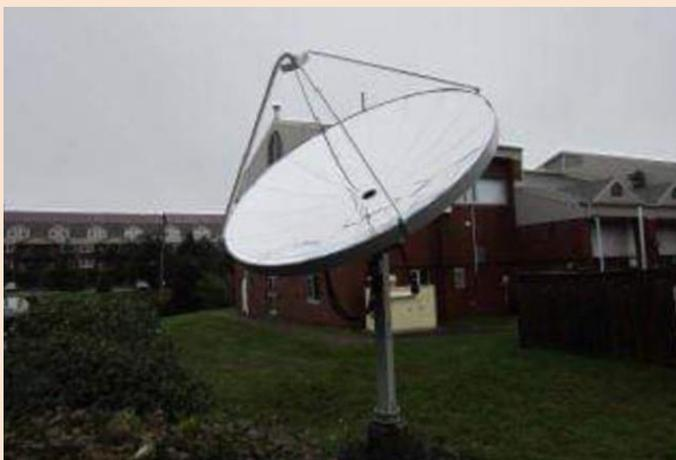
A lot of people drive by Fire Station #7 on dish Knightsridge Drive in Halifax wondering what the purpose of the large satellite is. As a matter of fact it is not a Satellite dish at all! It is a Solartron SolarBeam concentrated thermal solar collector that is intended to heat up hot water for use by the fire station. Have a look next time you drive by!
