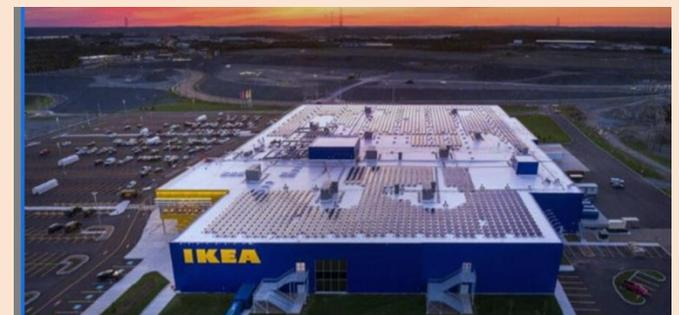
Solar Nova Scotia was pleased to offer a tour to Solar NS members this June of the new rooftop solar system at the Dartmouth Crossing IKEA. The system is currently the largest system in Nova Scotia at 850 kW. IKEA installed the system behind-the-meter to get around the current 100 kW net-metering cap in Nova Scotia. IKEA
