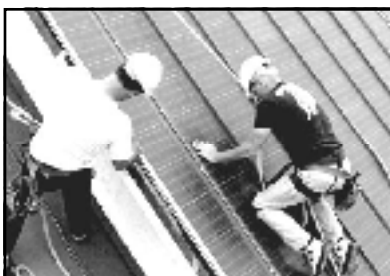
PV Metal roofing. (photo: www.toolbase.org)
