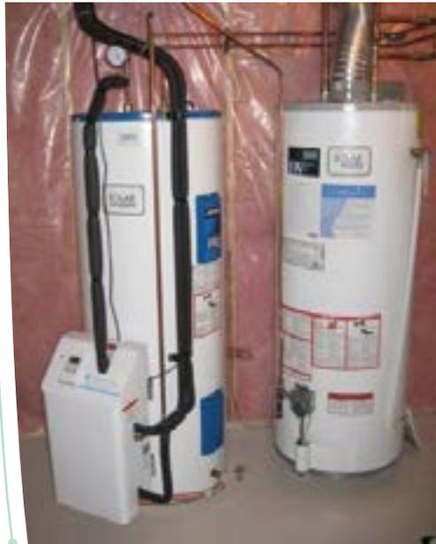
This is a very good match, as the PV-powered pump only runs when the sun is shining – which happens to be the time that the SDHW system is working.
